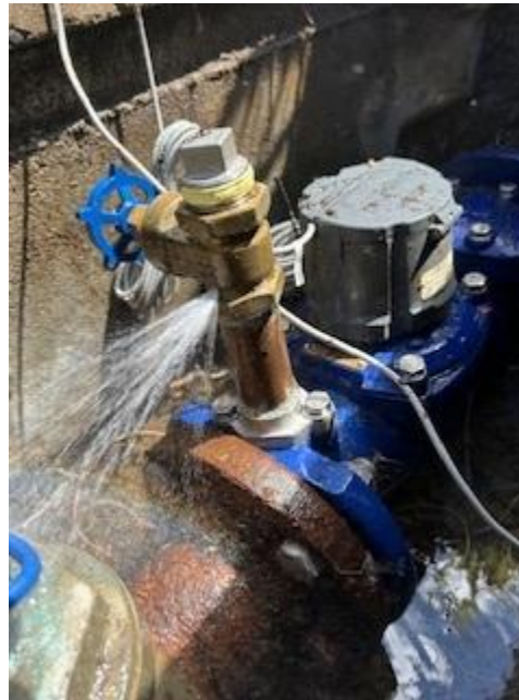
Small Valve Repair
