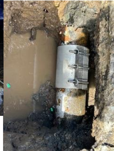
Main Repair Deskins St
